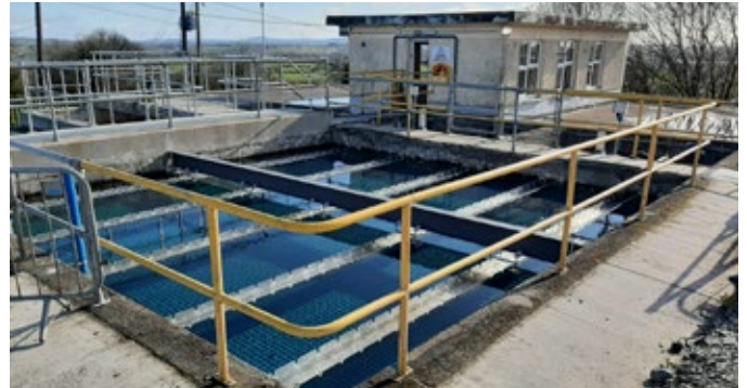
Plant is pictured, showing the upgraded clarifier in place.
